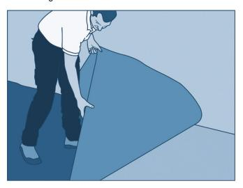
Installing textile floor covering with seam:
